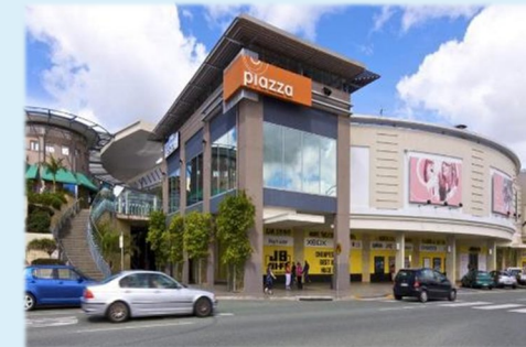
Hyperdome Shopping Centre Logan Equipment: ThyssenKrupp & Schindler Elevator Units: 3 Moving Walkway Units: 8
