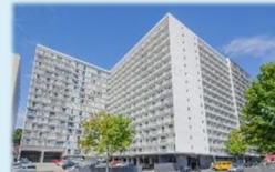
Zest Apartments Auckland Client: Pacific Properties
