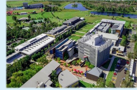
University of Sunshine Coast Sunshine Coast Equipment: Mixed Technologies Elevator Units: 29
