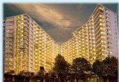
Volt Apartments Auckland Client: Pacific Properties
