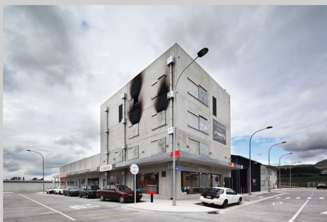
National Training Centre City Street
